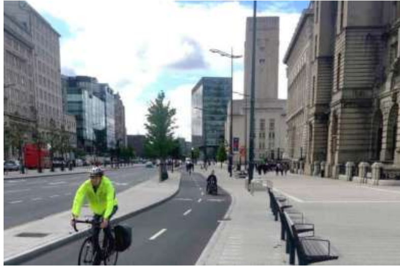
Image of a segregated cycle path and widened pavements on the Strand, Liverpool City Centre Source: LCRCA
