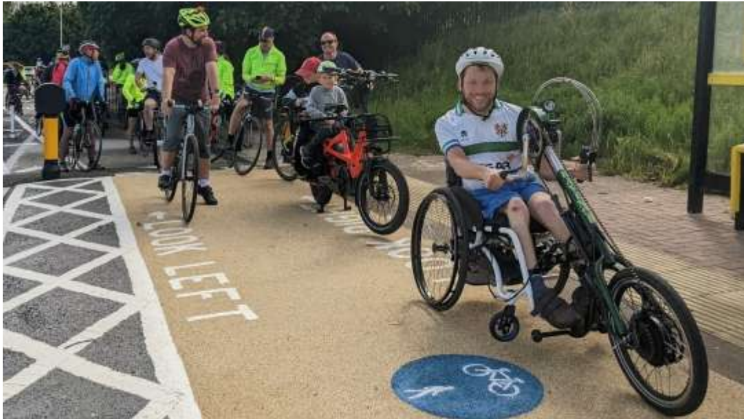
A fully accessible active travel route between Bidston and Moreton, Wirral Source: LCRCA
